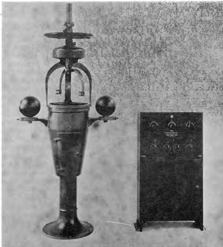
Kolster radio position finder; the first practical radio direction finder for shipboard operation, developed by Frederick A. Kolster at the Federal Laboratories in 1921 and manufactured by Federal. At the left is shown the loop compensator mechanism as attached to the standard ship's binnacle. The rod at the top supported a square rotatable loop antenna located above deck. The vacuum tube receiver employed with the direction finder is shown at the right.
